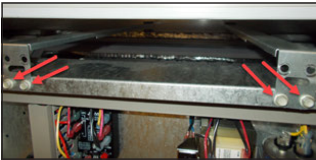
FIGURE 6 Remove Four Screws
