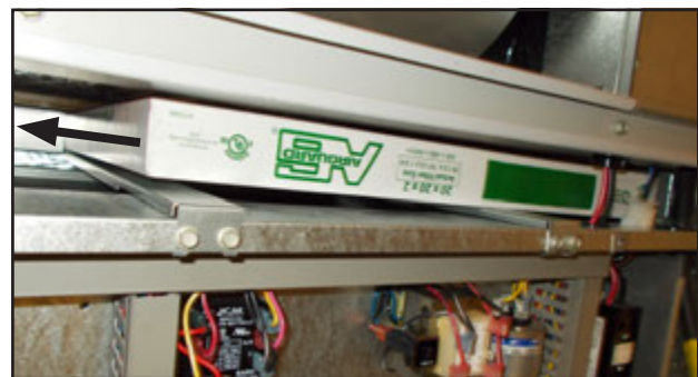
FIGURE 3 Removing Second Filter
