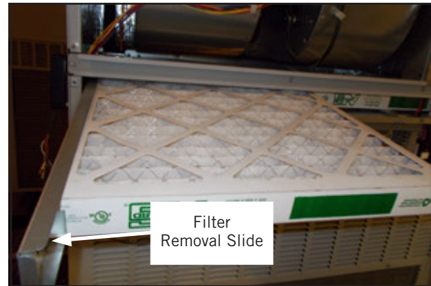
FIGURE 3 Removing Second Filter
