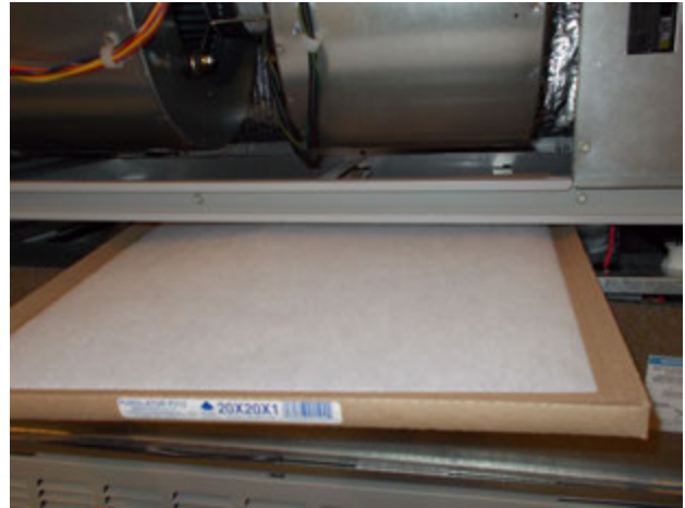
FIGURE 9 Install Left 1" Filter
